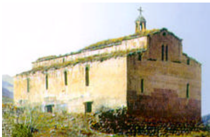
The Tzitzernavank Monastery, St. Gevorg Basilica, V century AD
